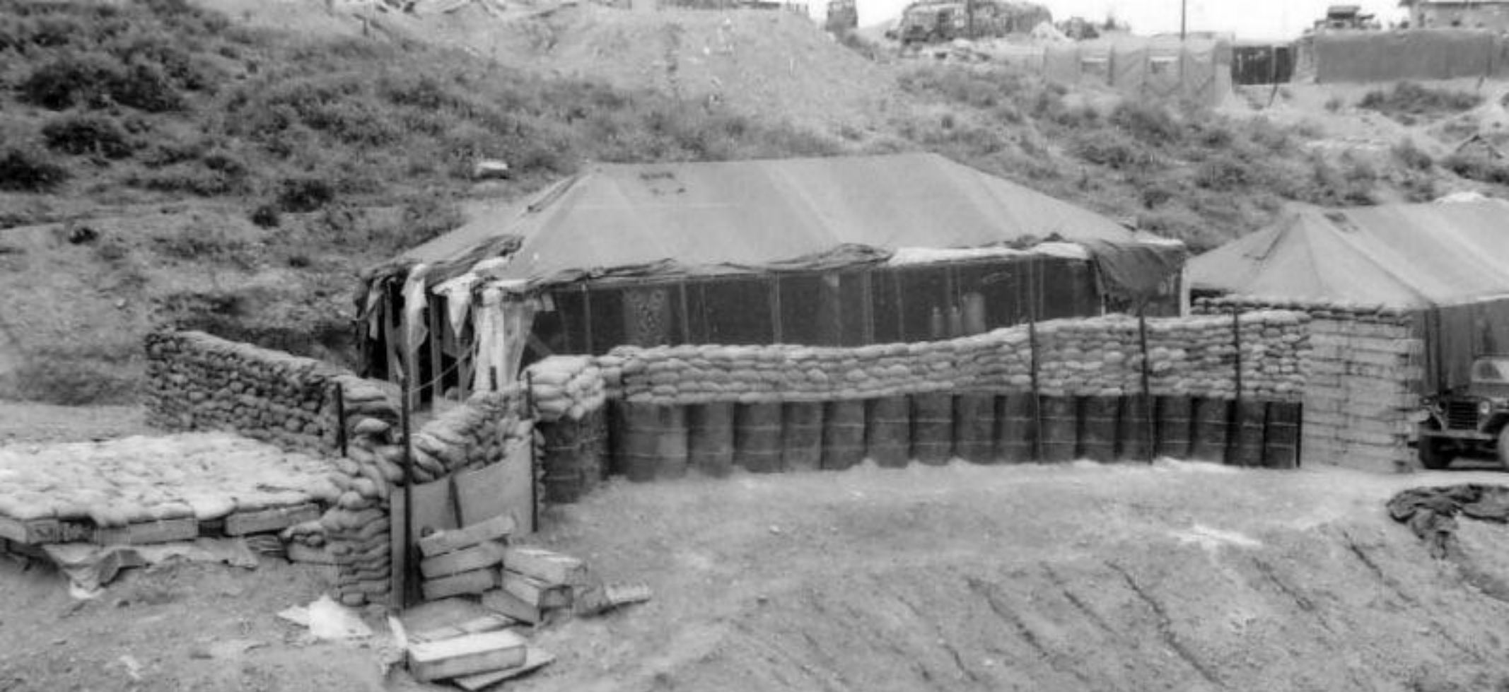
B and C Btry supply tents in the ravine at LZ Sharon, with the BN CO's hooch at the upper right. July, '68
